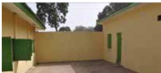
Renovated Boys Hostel at School for The Blind, Deaf and Dumb, Yelwa, Bauchi by our Bauchi staff
