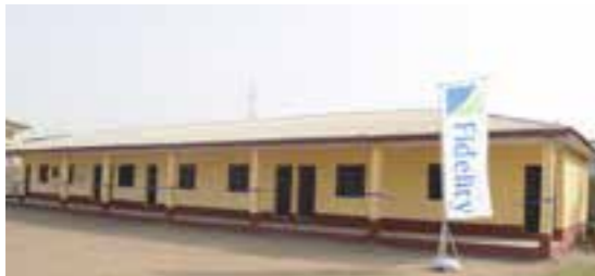
The renovated and equipped block of classrooms at Ibafo Primary School, Olodi, Apapa, Lagos by our Apapa branch staff
