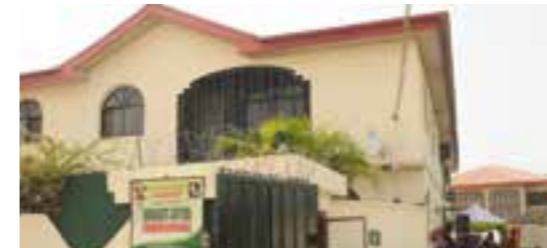
The renovated Sought After Motherless Children's Orphanage home at Ajah. Executed by Head Office staff
