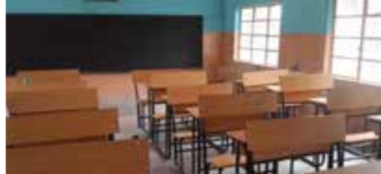
Renovated blocks of classrooms in Zaria Childrens School by our Zaria staff
